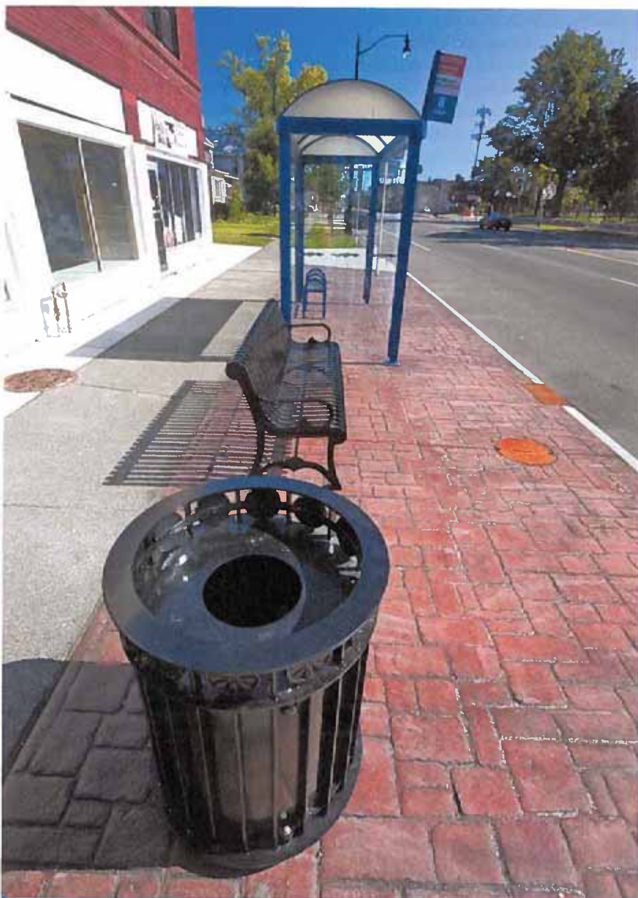
All sidewalks of the project were replaced using an exposed aggregate mix, which lends a historic texture to walkways. Snow-storage strips were replaced with red-tinted concrete with a block stone pattern and gray release.
